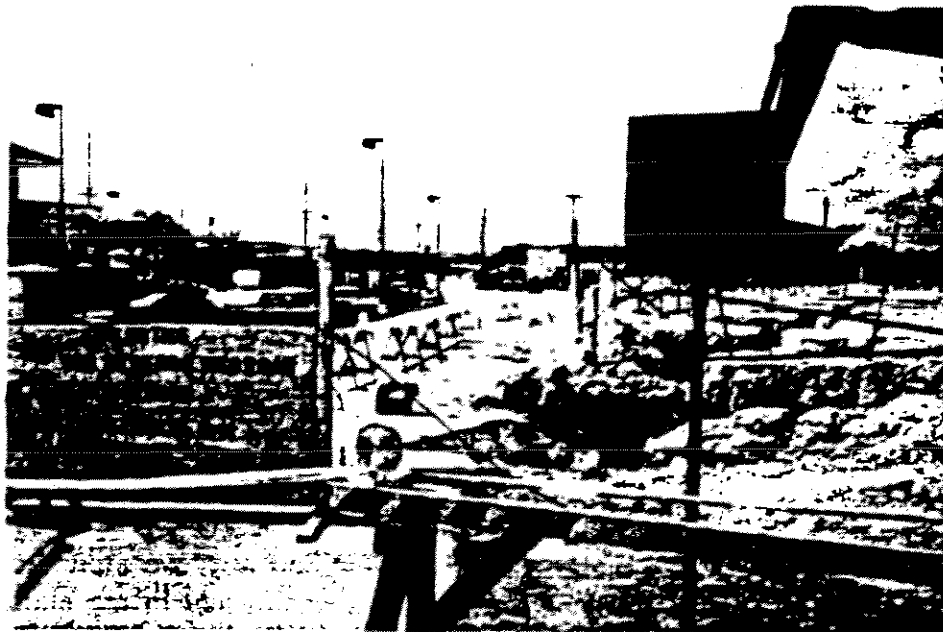
Figure 5. Cold Storage road looking south from Route 16 shows the right lane closed and construction in process in the roadway. (Office of Inspector General photograph - December 19, 1991)
